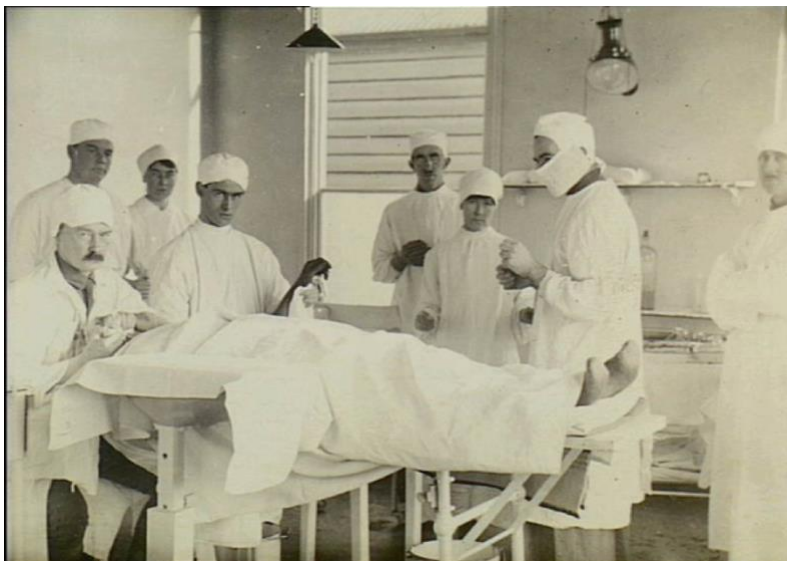
The operating theatre and staff at No 3 Australian Auxiliary Hospital. Staff members, from the left, are Captain (Capt) South, Capt J. Lambert, Sister D. Rogers, Private (Pte) H.J. Jones, Capt K. Rae, Sister Kennedy RRC, Lieutenant Colonel V. Hurley CMG, Capt Fay MC and Bar. Pte J.B. Leslight is on the operating table. January 1919 England, Kent, Dartford. Photo: Australian War Memorial
