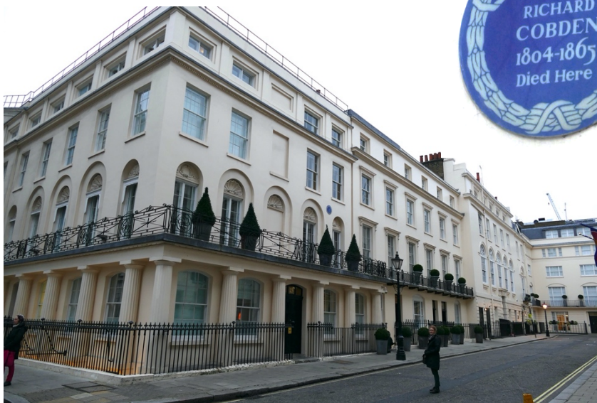
The apartment with the Blue Plaque (insert) in Suffolk Street, London, where Richard Cobden died. Photos: Euan McGillivray 2016
