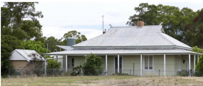
From his step-granddaughter's description, I believe this to be the mudbrick house built by Benjamin Blunden at Amphitheatre Victoria. The mudbricks covered over with fibrocement sheeting at a later date, apart from the out building to the left. Photo: Euan McGillivray 2021
