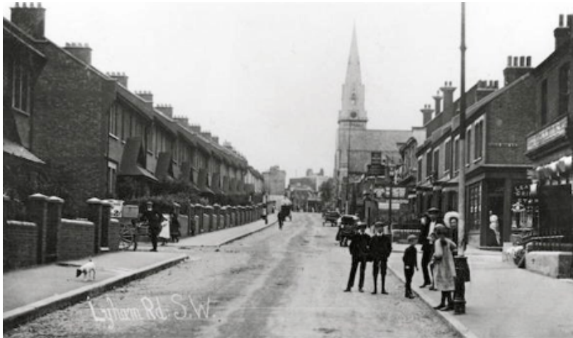
Lyham Road, Brixton, looking south. Nelson's Place where the Fowles family lived, would have been a row of houses on the left, demolished and replaced by the ones seen here in c1905. Source: London Borough of Lambeth
